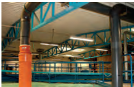
Sewage water treatment plant
